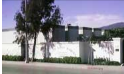
The Charles Meyer Desalination Facility serves the City of Santa Barbara
