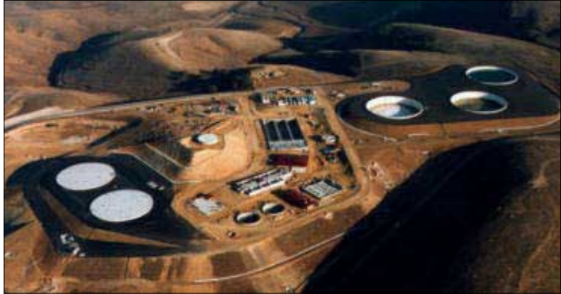
Polonio Pass Water Treatment Plant
