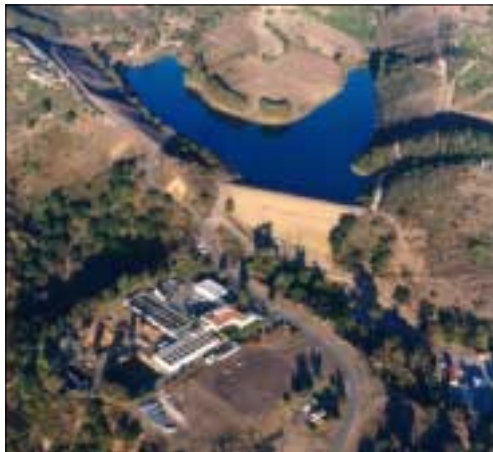
Lauro Reservoir and the Cater Water Treatment Plant
